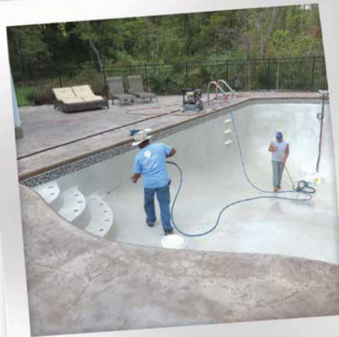
drain and clean pool
